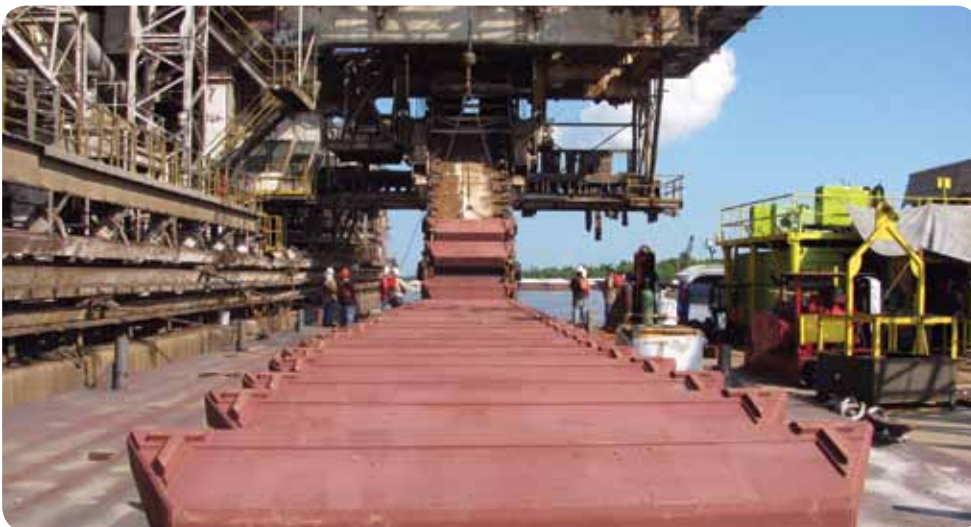
New buckets being installed on barge unloader.
