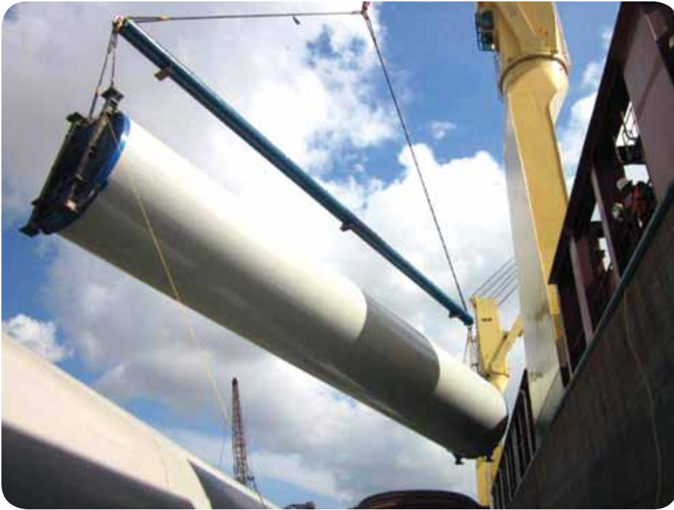
Associated transferring windmill tower sections from ship-to-barge in calm water slip at the Port of St. Bernard.
